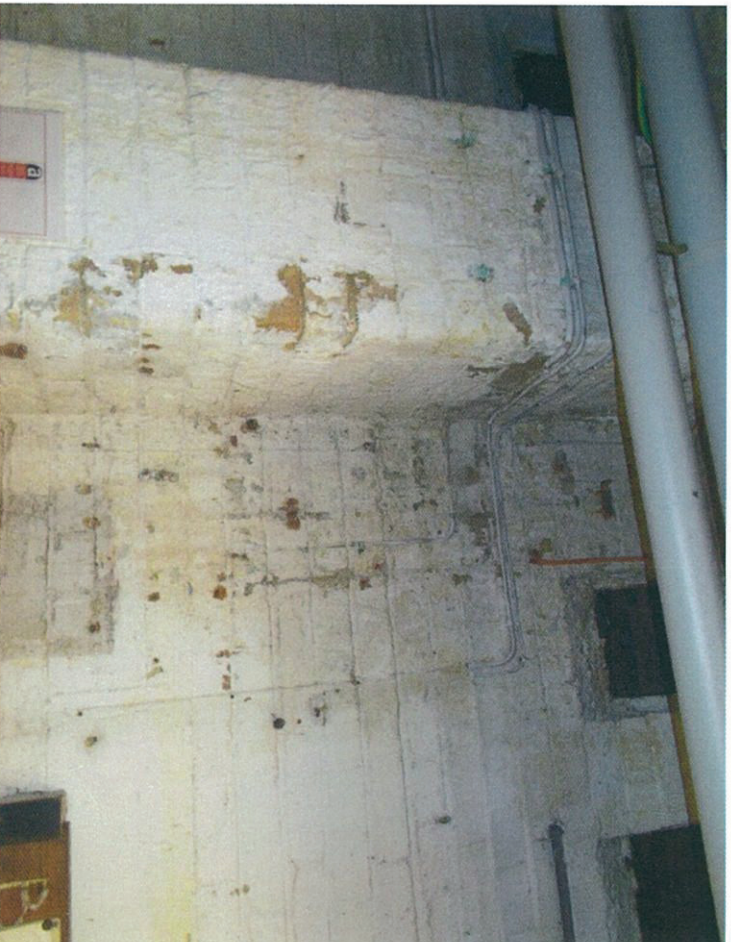
Photo 17 Corrosion to Embedded Steel within Basement Ceiling
