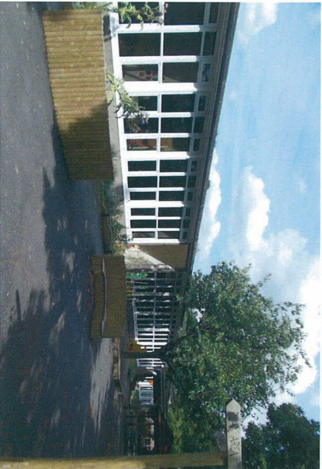
Photo 10 General View of South Wing
