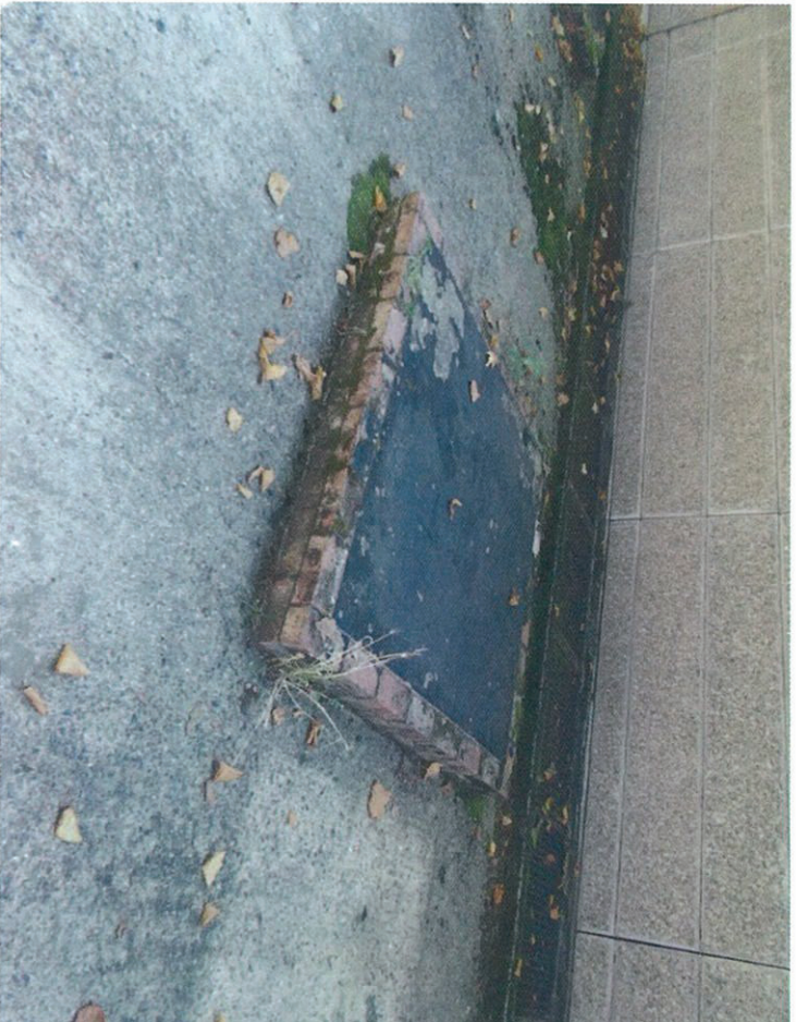
Photo 5 Basement Penetrations to North Hard Standing
