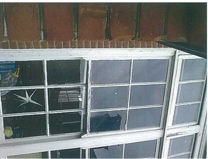
Block A – Upper Windows
