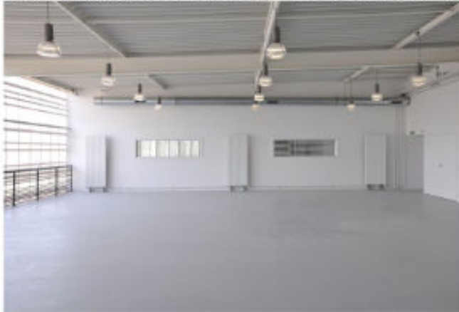
LOCALISED CLEARANCE OF REDUNDANT SERVICES TO MAKE GOOD AND REFURBISH WITH HIGH QUALITY MATERIALS.
