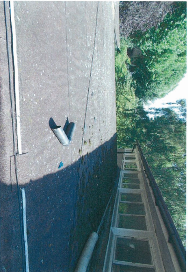
Photo 6 Example Condition of Roof Covering
