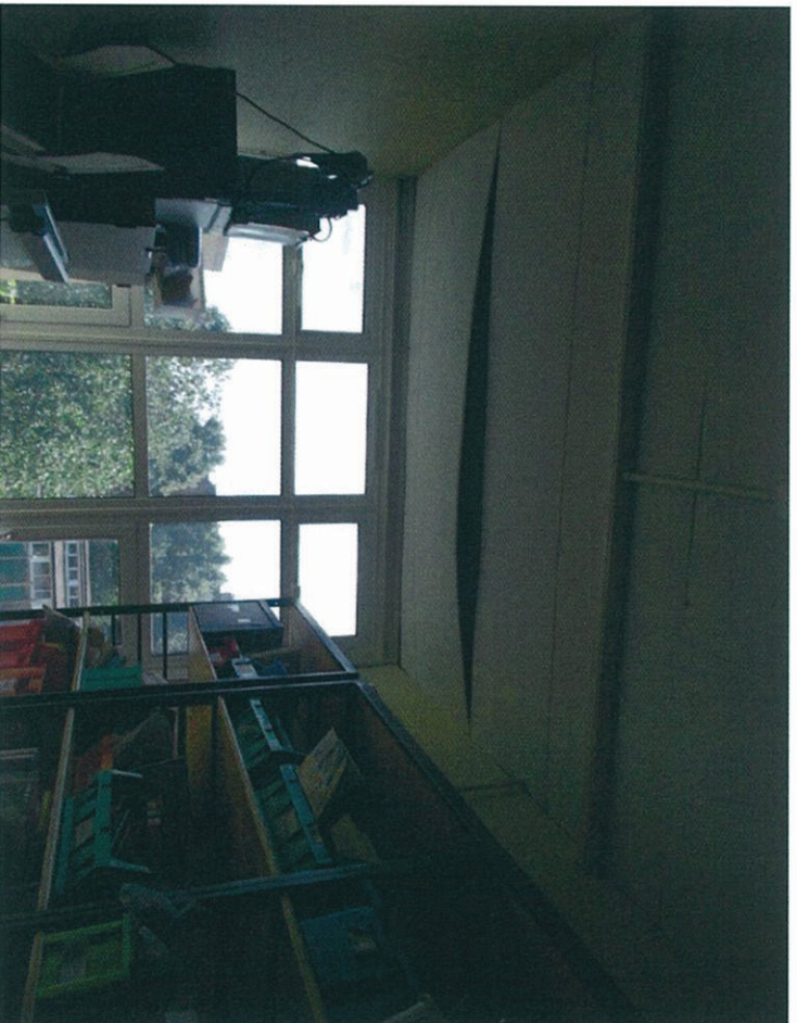
Photo 15 Failing Ceiling Boards
