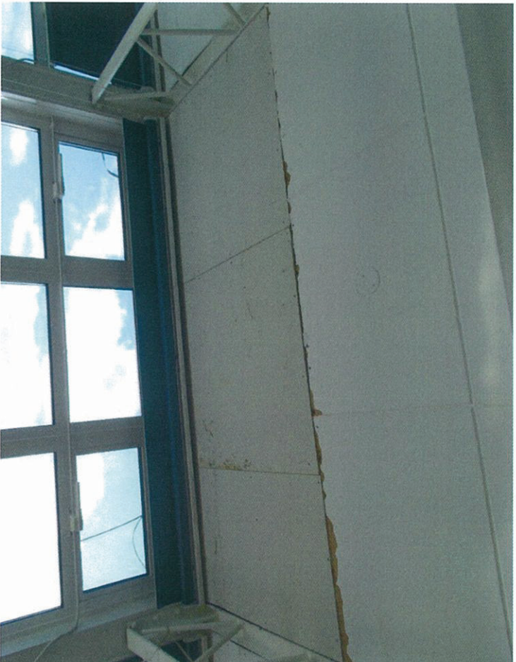
Photo 15 Failing Ceiling Boards
