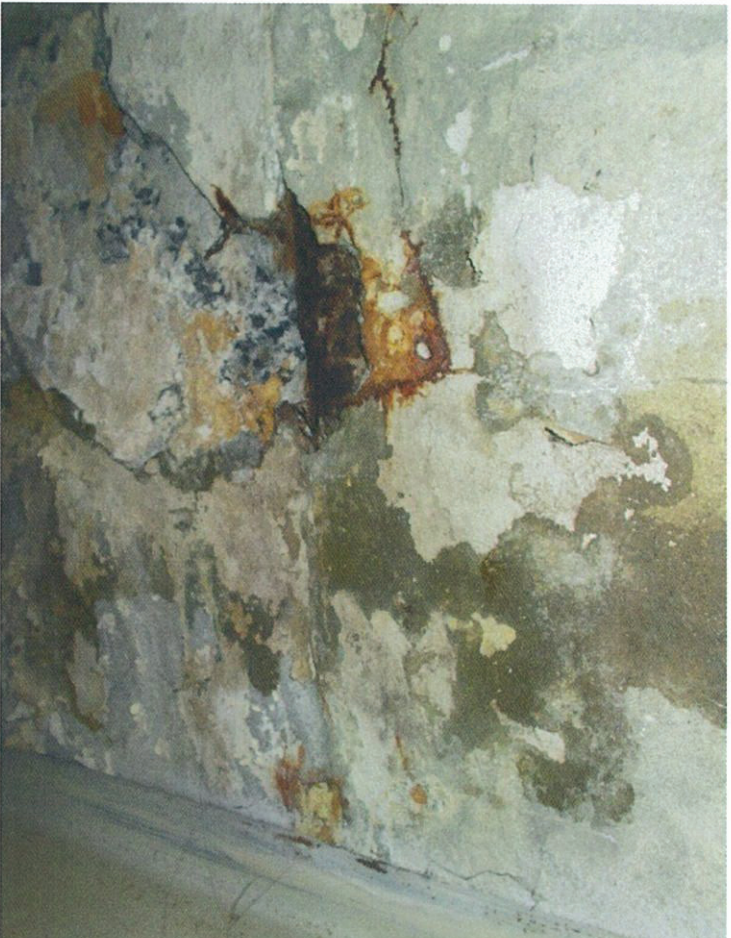
Photo 17 Corrosion to Embedded Steel within Basement Ceiling
