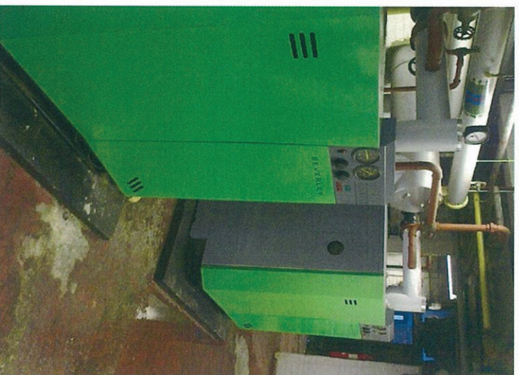
Photo 19 Basement heating boilers, water ingress
