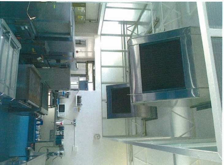
Photo 25 Main kitchen, extract ventilation to all electrical catering equipment
