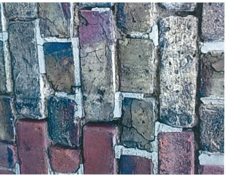
Block A – Brickwork
